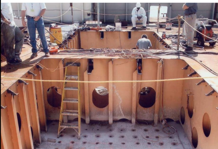
**Top:** Removing a large section of the ship's 9-foot-thick ballast was necessary to reduce its weight.
