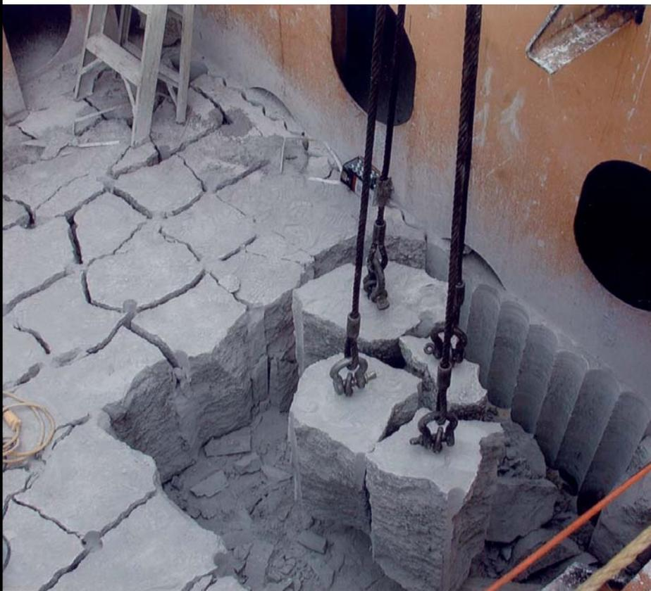
Top: Line drilling around the perimeter created room for the concrete to shift during the breaking process.
